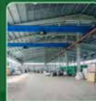
Warehouse & Cold Storage
